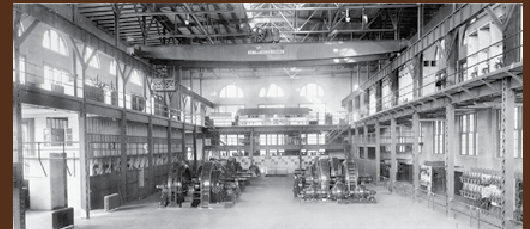
Photo courtesy of Avista. The substation's large, open interior allowed various equipment configurations and dissipated machine-generated heat. Equipment in this 1913 view provided AC and DC power at various voltages.
