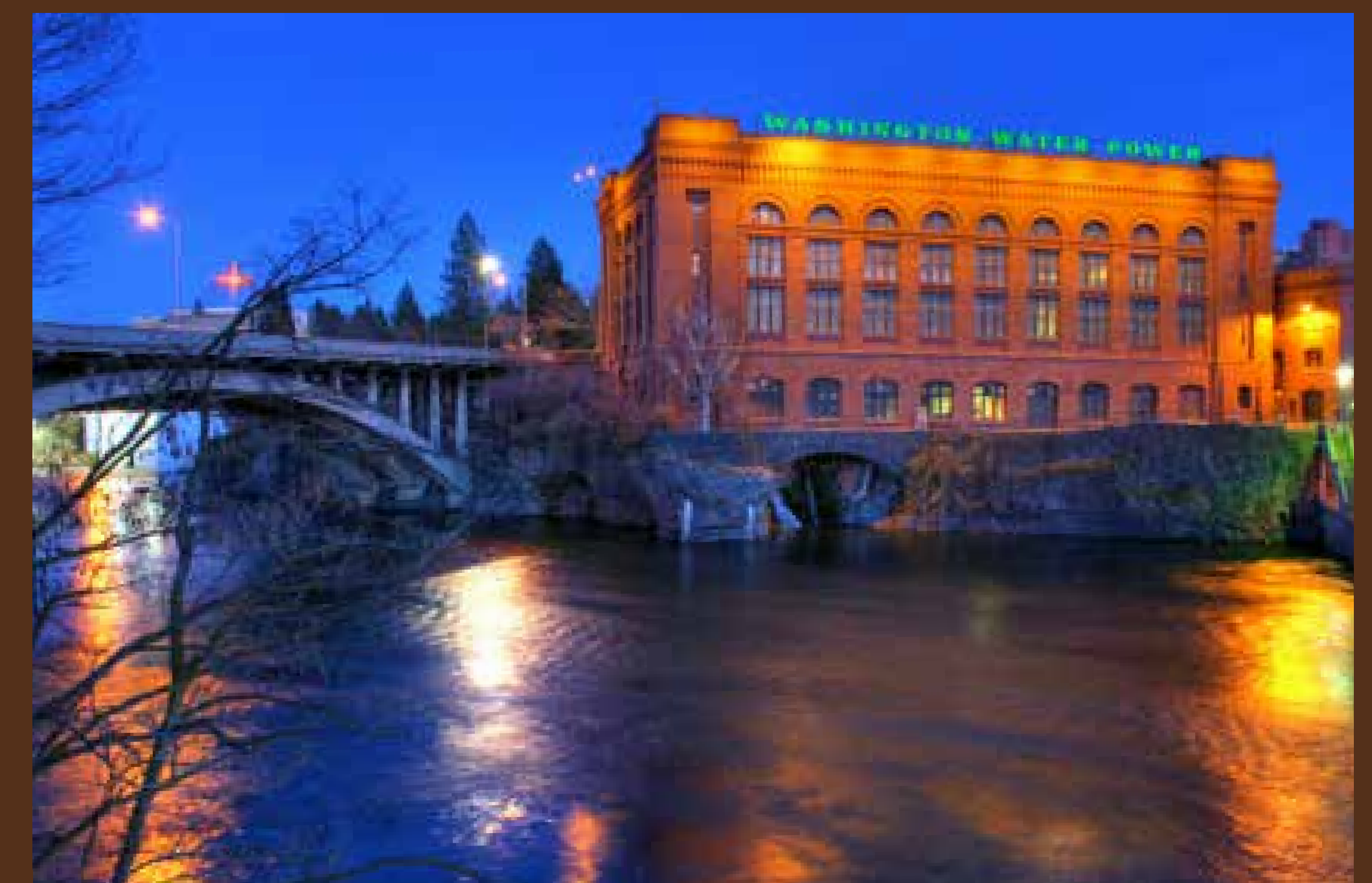
Photo © 2009 John D. Moore, CPP. Avista's Post Street Substation has been an integral part of Spokane's waterfront since 1909.
